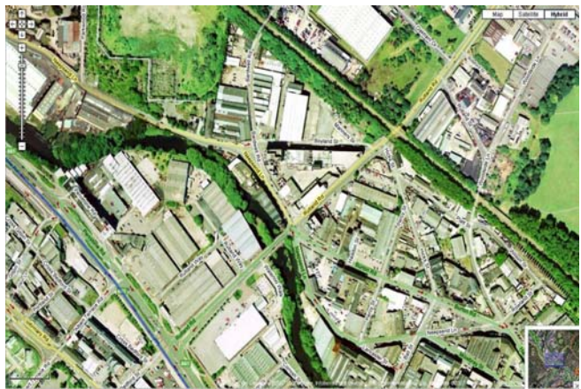
Figure (20/ b): Linear shape of urban trees, Upper Hanover Street, Sheffield, UK.
