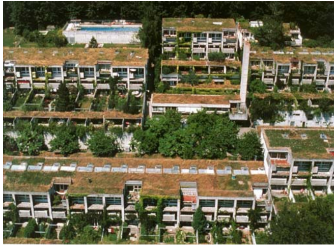
Figure (20/a): A combined array of green roof with a remarkable block back yard with roof garden affect the local urban climate and break the heat islands chain regarding the canyon geometry, canyon trees, slope with orientation and housing types.
