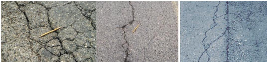
Figures (2): shows the different types of cracks; alligator (fatigue) cracking, longitudinal cracks and non-wheel path cracks.
