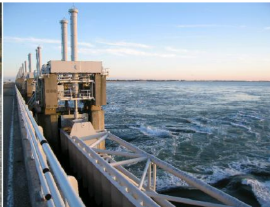
Fig 4: Vertical Lift Gates (Delta Project).
