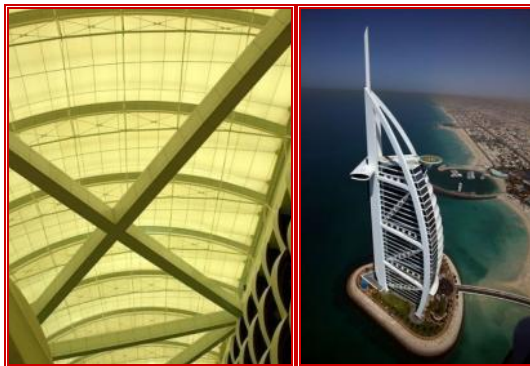
Figure-1: Membrane reduces glare and allows diffused lighting into atrium Burj Al Arab
