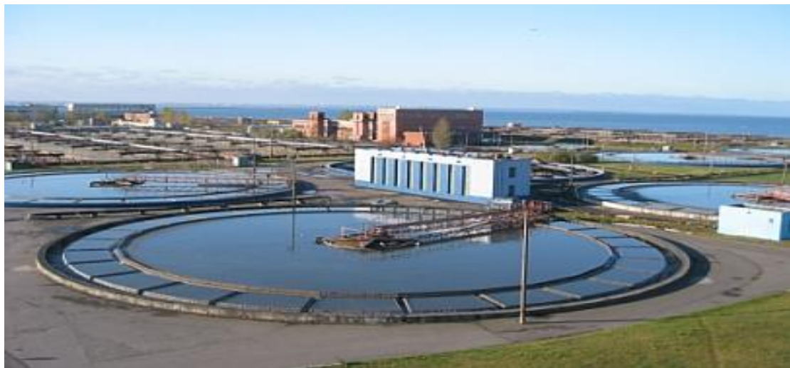
Figure 5: Shows Phosphorus Removal Plant in Russia.
