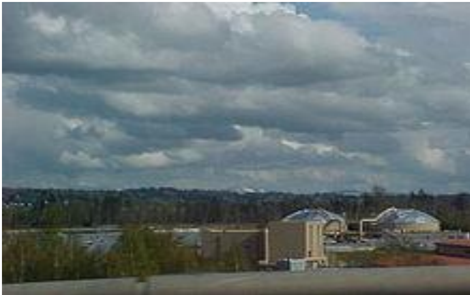
Figure 3: Shows Sewage plant and Lagoon in Everett Washington.
