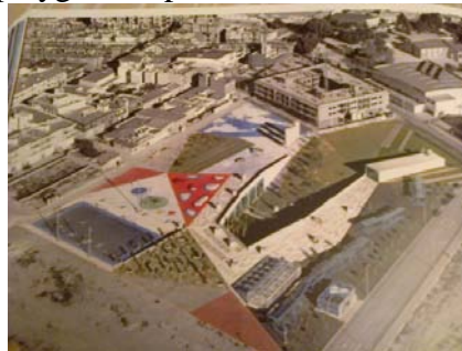
Fig (3) an aerial image of the Municipal library and reading park in Torre Pacheco Spain [10]
