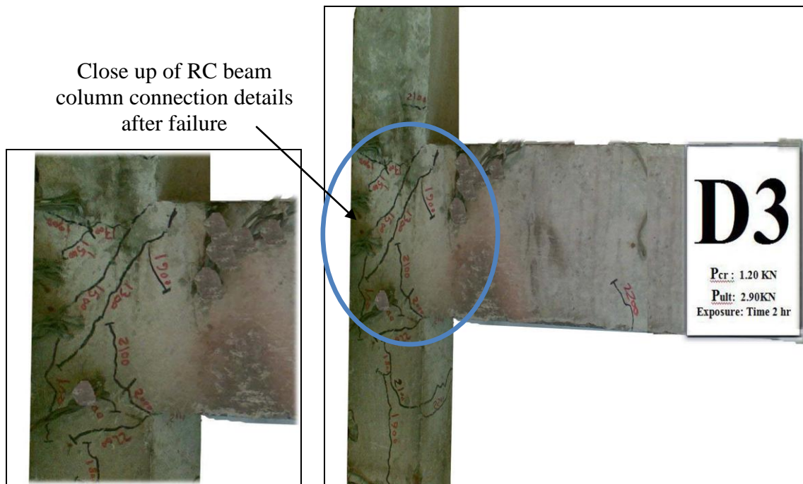
Figure (14) Crack Pattern and modes of failure of RC Specimen D3 at 600°C for 2hr
