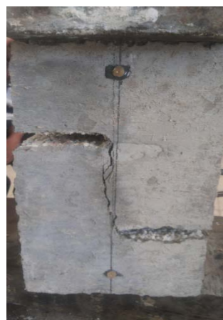
Figure (9) Crack Pattern and Shape of Failure of Specimens
