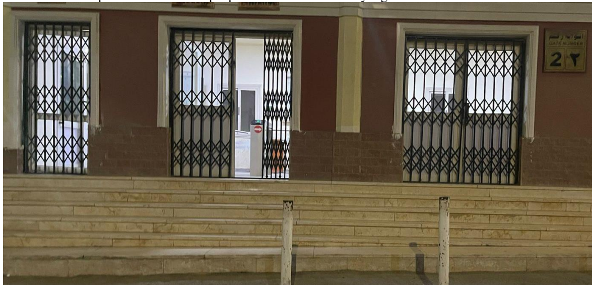
Figure 2 (gate 2) six stairs.
