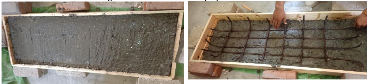
Figure 5. Cast of reinforced concrete slab
