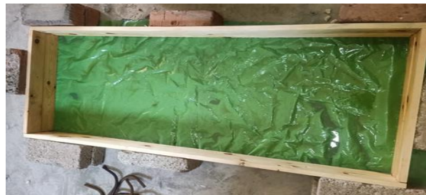
Figure 4. Formwork used to prepare the slabs
